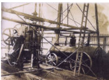
Victorian Coal Mining Company Diamond Drill & the Helena steam portable boiler at the Red Bluff exploration site 1893-1897
